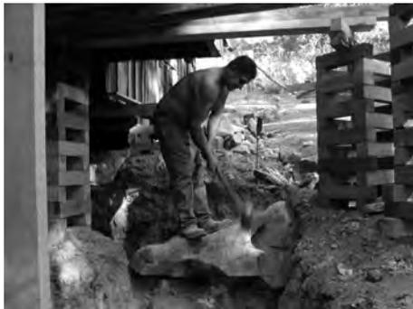
Hired help: Mario demolishes the large rock where the walls will stand. Around him is the 4X4 cribbing used to jack up the house.
