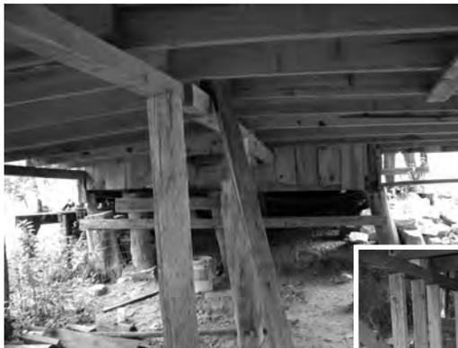
Left: After a decade on the original posts, the warping and bending are obvious. The outside corners the house had settled over 25 centimeters. Below: The fieldhouse sitting on new block foundation walls, Spring 2009.
