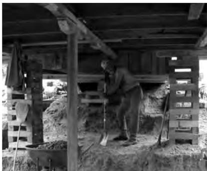
Ediger operating the excavator on the helper's day off. About 120 centimeters of material had to be excavated just to get to floor level on the high end. The bottom of the footer was another 30 centimeters lower.
