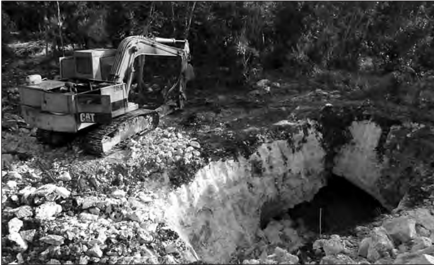
Figure 2. Recent example of cenote enlargement using heavy machinery. In this case, the goal of the landowner was to create an open-water pool to attract paying snorkeling tourists. Robbie Schmittner.
