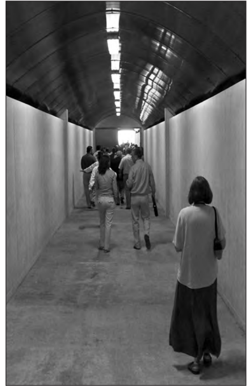
The new entrance tunnel.
