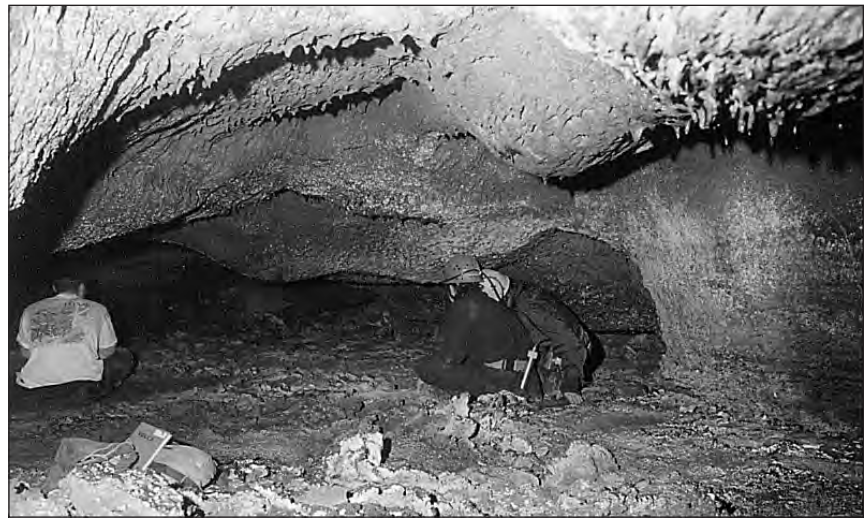
Figure 10. Chamber in H-74, showing sagged parts of roof.
