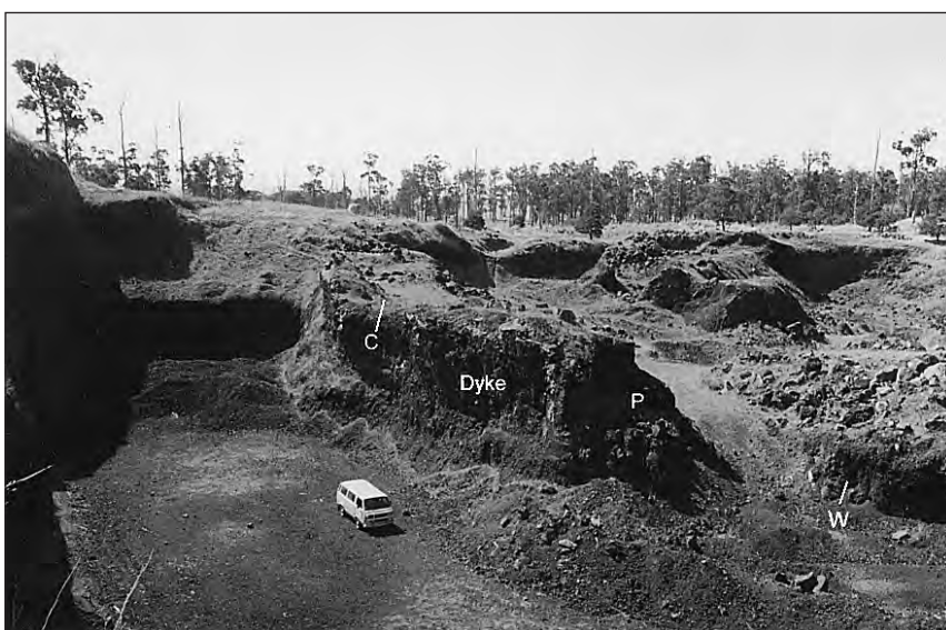
Figure 1. View of Mt. Fyans Quarry, looking north towards the large dyke. C = cave, P = Pipe, W = Witch’s hats.
