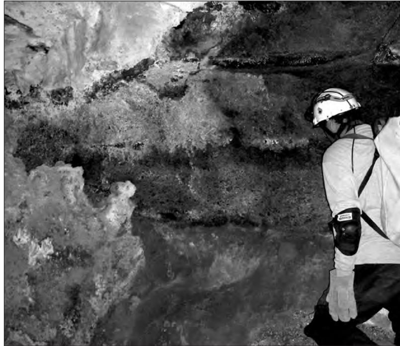
Tephra layers behind lining, evidence of thermal erosion.
